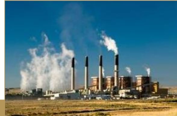
Cochise Power Plant, Arizona
